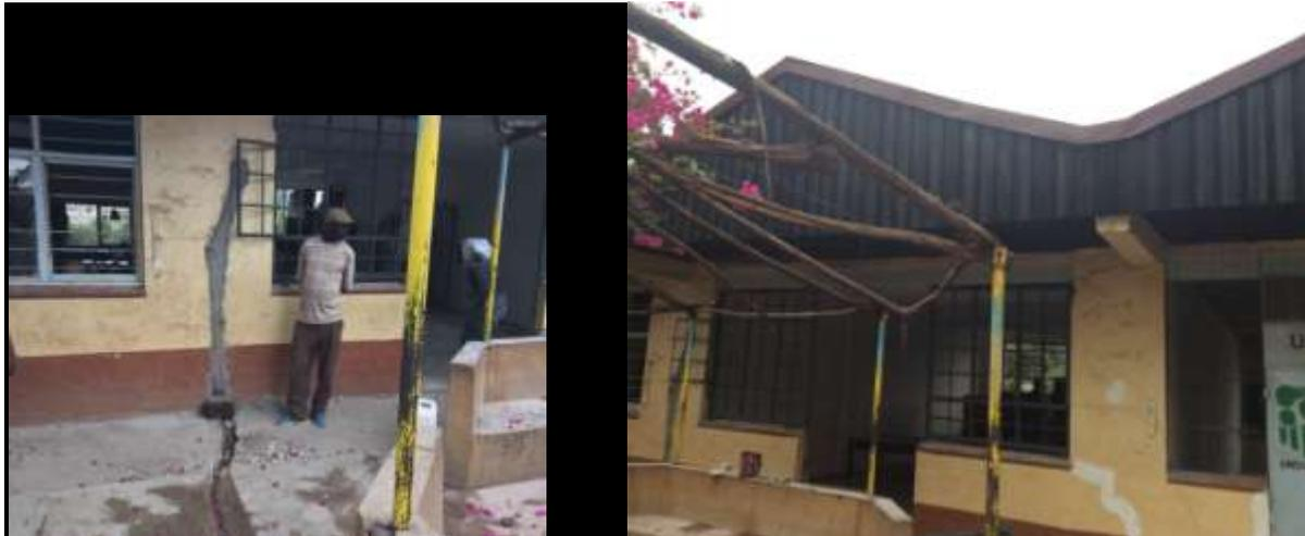
All the old wooden windows were removed and replaced with new aluminium windows, complete with burglar proofing. Skimming with gypsum powder was done for a smooth wall finish and brand new paint was used to give it the new look that it has now.
