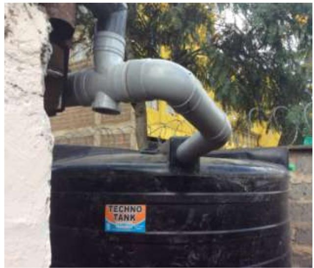
In phase two of the project, this water tank will also be connected by pipes to other smaller water tanks that will be mounted onto a slab that will be created above the toilets. A water pump, complete with a pressure control unit was purchased and has been connected to this main water tank so that when water runs out from the main grid under the Nairobi City County (and these shortages are quite frequent) , the harvested rainwater can serve the abolition block and hand-washing sink area.
